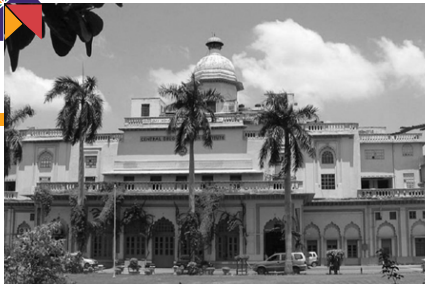
Kaiserbagh Palace, Lucknow
